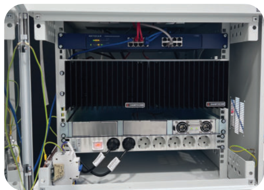
Danphone's VHF Transceiver operating in the marine VHF band mounted in rack.
