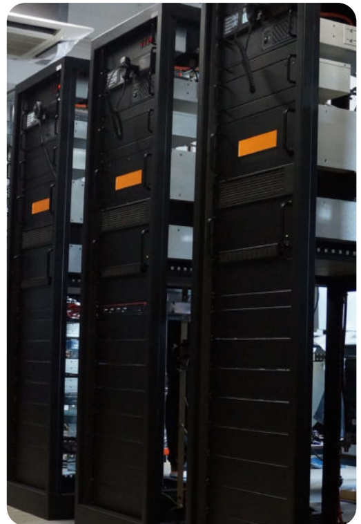
Multiple-racks for large scale systems.
