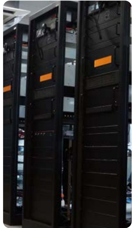
Example of multiple-racks for large scale solutions.
